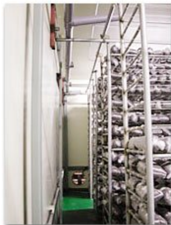
Air-inlet duct and air-outlet fan
