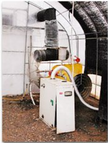
Ancillary room Boiler and fan for flowing hot wind
