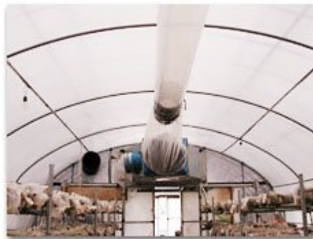
Growing room Duct, left (black) for hot air and center (plastic pipe) for cool air
